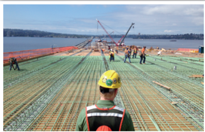
Reinforcing Steel being placed by Rainier Steel on the SR 520 Floating Bridge Project in Seattle.
