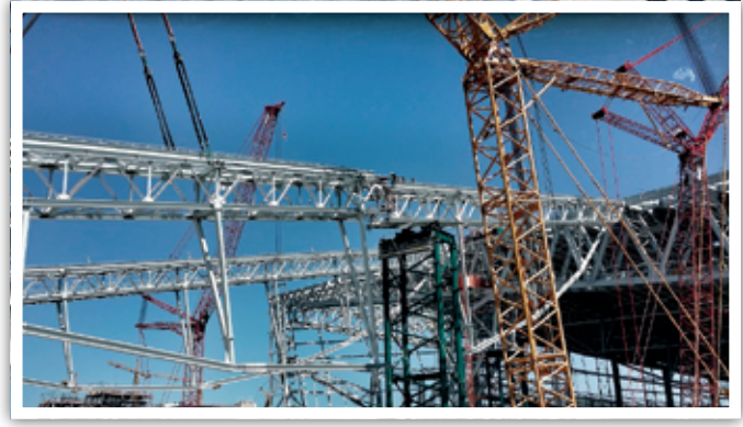
Iron Workers Local 512 (Twin Cities, Minn. and St. Paul, Minn.) and Danny's Construction Company topped off the U.S. Bank Stadium for the Minnesota Vikings in 2015.
