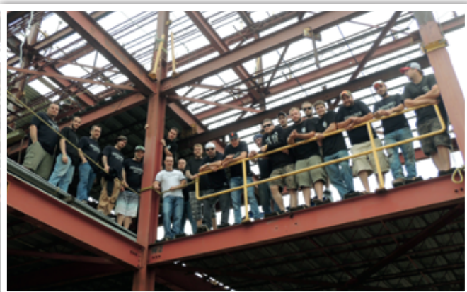
Local 721 (Toronto, Ontario) ironworkers working on the Regional Training Center in Toronto.
