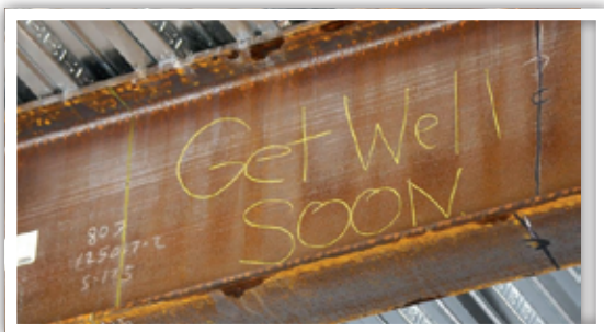
Iron Workers Local 396 (St. Louis) left this note for St. Louis Children's Hospital patients while erecting the structure.
