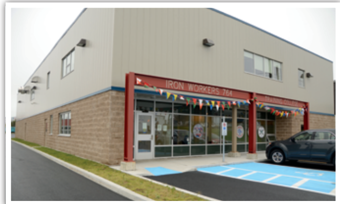
The Local 764 (St. John's, Newfoundland) Training Center officially opened in September.
