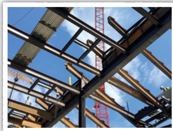
Local 5 (Washington) ironworkers detailing iron for the MGM Grand Casino at National Harbor in Washington.
