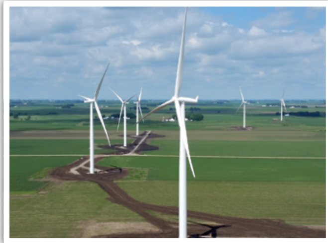
Iron Workers Local 21 (Omaha, Neb.) helped to build the Highland Wind Farm in Primghar, Iowa. It is the state's largest wind farm, with 214, 2.5 mega watt general electric turbines.
