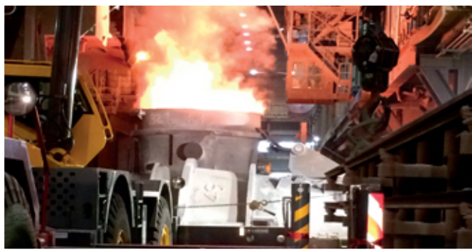
Iron Workers Local 395 (Hammond, Ind.) and Pangere Corporation worked diligently to maintain 100 percent safety compliance on this project for ArcelorMittal.
