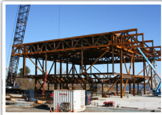
Construction on the Edward M. Kennedy Institute for the United States Senate.
