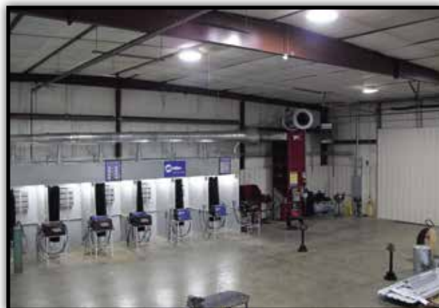
New welders and fume extraction system at Local 577 training center
