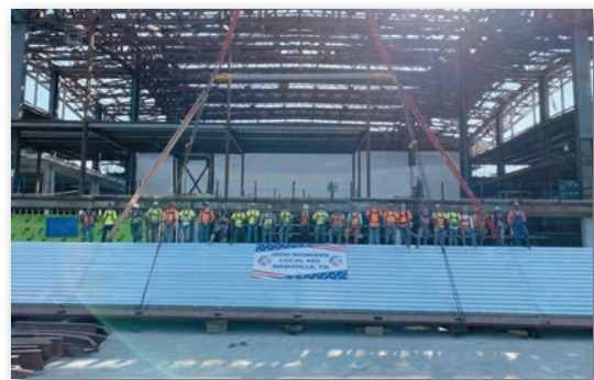
Iron Workers Local 492 (Nashville, Tenn.) Topping Out Nashville Airport Project
