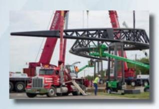
Superior Steel Erectors lifting Lenexa Gateway signal truss in Lenexa, Kan.
