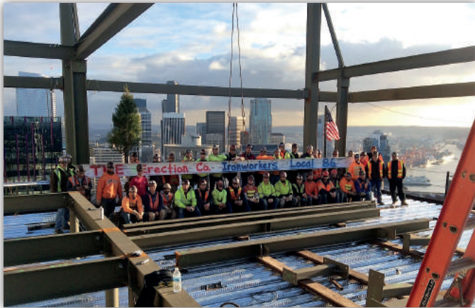
The Erection Co./Local 86 (Seattle) ironworkers topping out on the Amazon Project
