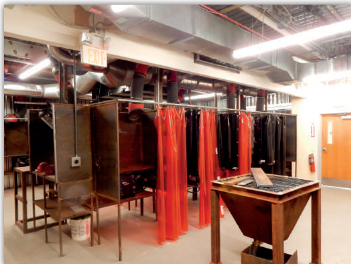
Welding Shop in the new Local 15 (Hartford, Conn.) training center
