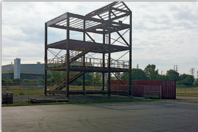
Training structure purchased with grant money for Local 9 (Niagara Falls, N.Y.)
