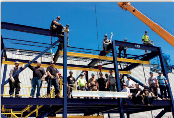
Apprentices training at the Local 736 (Hamilton, Ontario) training center
